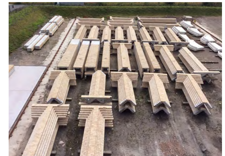
Modular facade components
