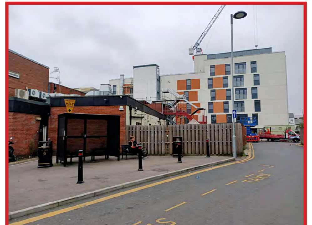
Compromised back conditions behind the High Street Wellstones
