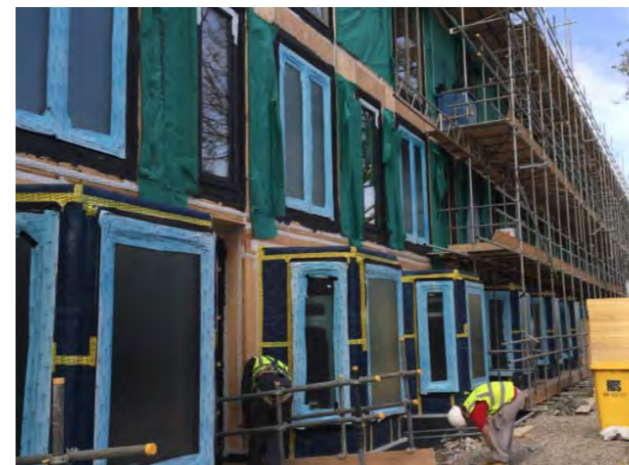
CLT components being assembled on site
