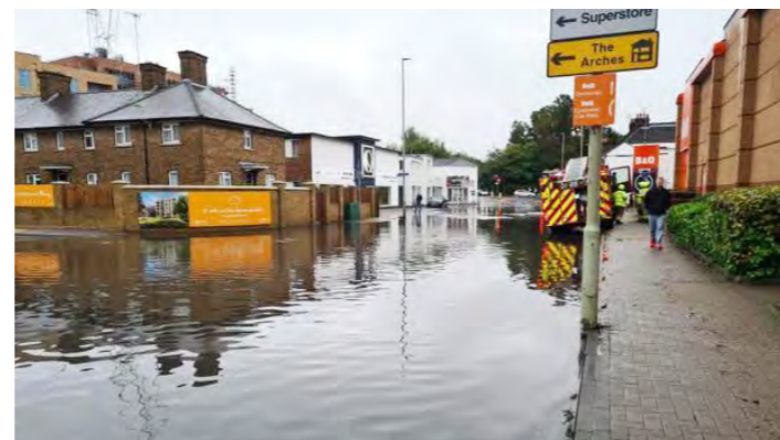
Flooding on Lower High Street, Watford forced multi-day street closure. 2014
