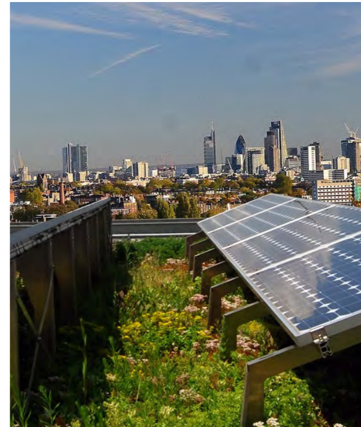
Coordinated rooftop space for greening and PVs London
