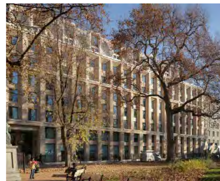
Modular construction Cartwright Gardens, student accommodation Maccreeanor Lavington
