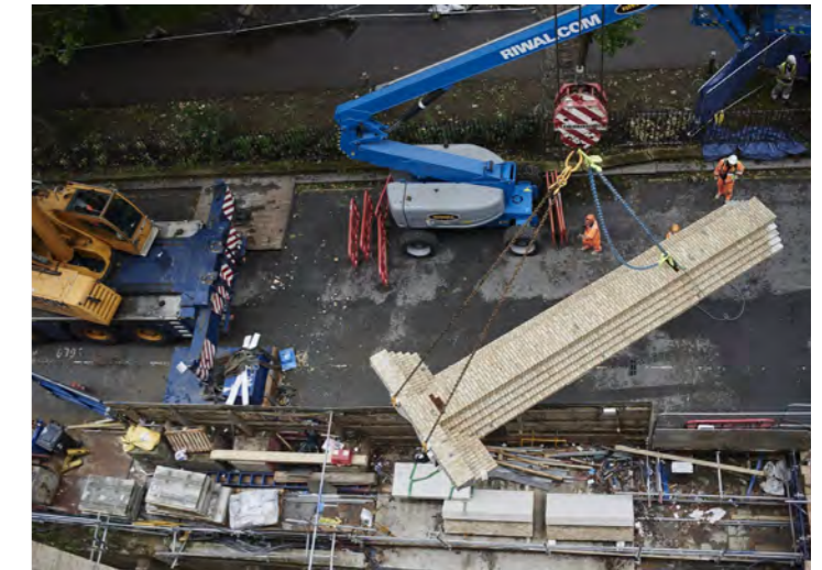
Modular facade components being positioned on site
